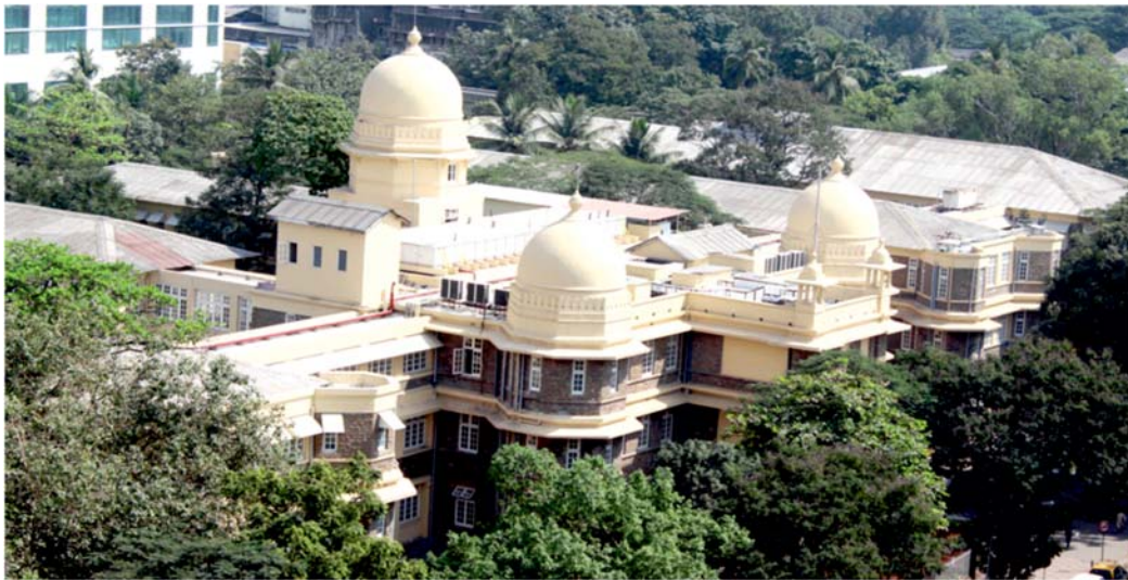
Aerial View of BJWHC.
